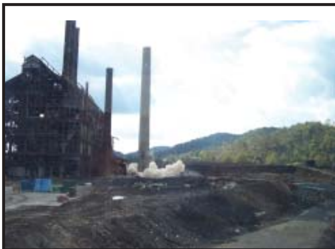
200+ ft concrete stack implosion.
