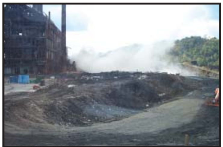
200+ ft concrete stack implosion.
